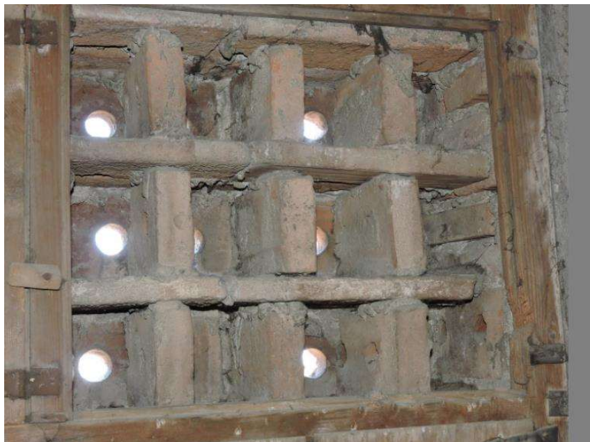
Figure 12: Patterned brickwork nesting cells for sparrows, seen from the inside
