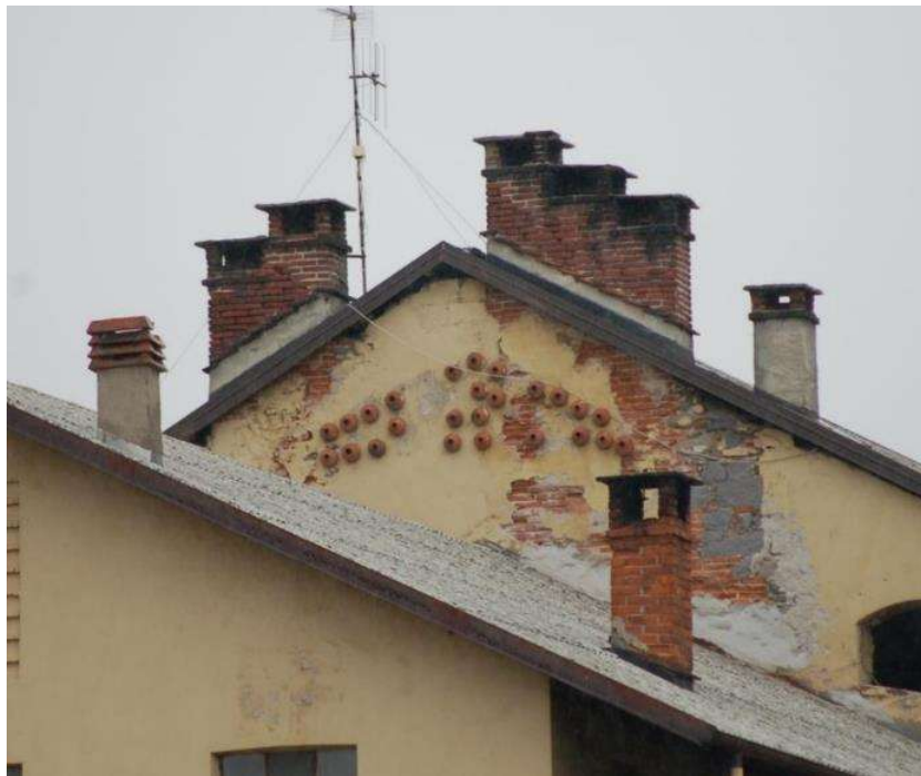
Figure 2: A cluster of bird pots on the wall of a dwelling (Biella, Italy)
