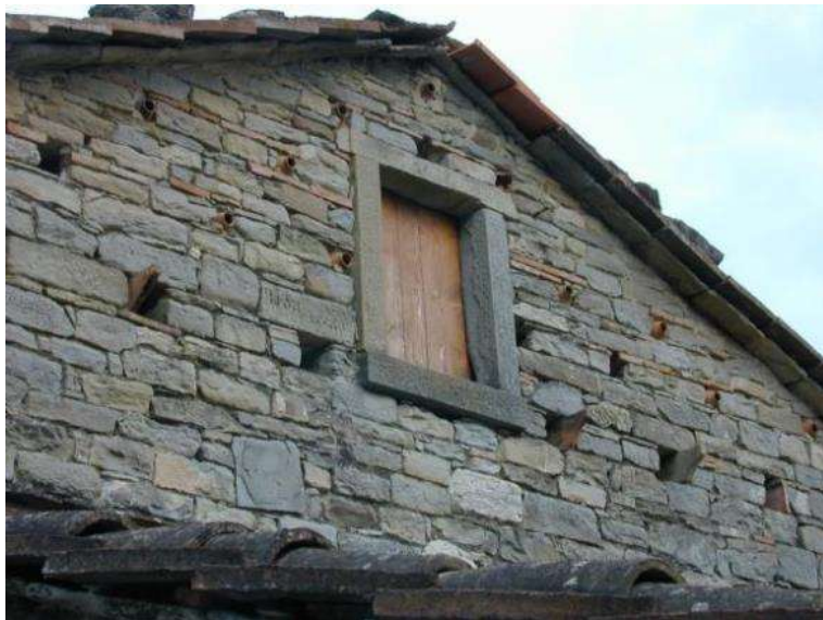
Figure 9: Swift pots partially embedded in the walls of a dwelling, Appennine of Romagna, Italy Photograph © Mauro Ferri
